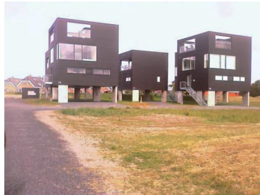
Figure 15: Summer houses in the port area of Rømø. The lower floor may not be used for living in, since the height from ground to first floor is insufficient for use as living space. Source: Flemming Kondrup.
